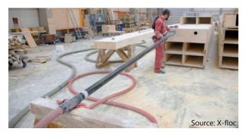
The blow-in openings are created into the frame. The rigid pipe allows a higher raw density to be introduced and also compacted. In addition, the distribution in the cavity is very even.
