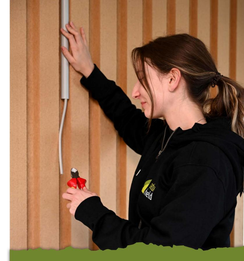
With naturheld 140-Install, installers can reduce installation time on site. The solid wood fibre insulation board is factoryfitted with pre-milled installation channels.
